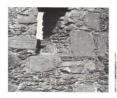
The original lime-mortar, as seen where not obscured by later pointing or rendering, contained calcined sea—shells, and is of a very resistant quality, as noted by Lamplugh (The Geology of the Isle of Man, 19O3,p. 566).
